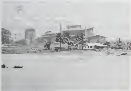
Iron-ore washing plant at Buchanan, Liberia Bo Dahlin—Ostrman Agency
